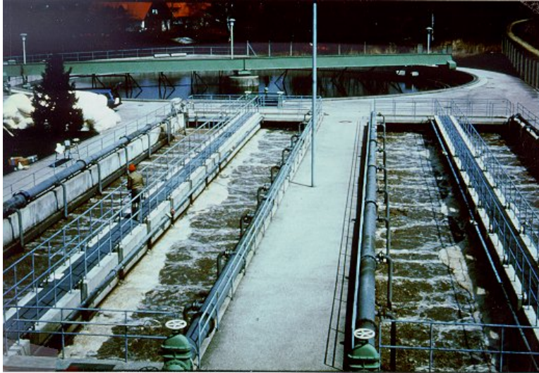
Figure 18 LinPor-CN™ Plug Flow Reactors at Freising DEU
