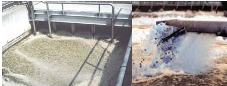
Figure 3 high “G” turbulence zone (left) impingement plate (right)
